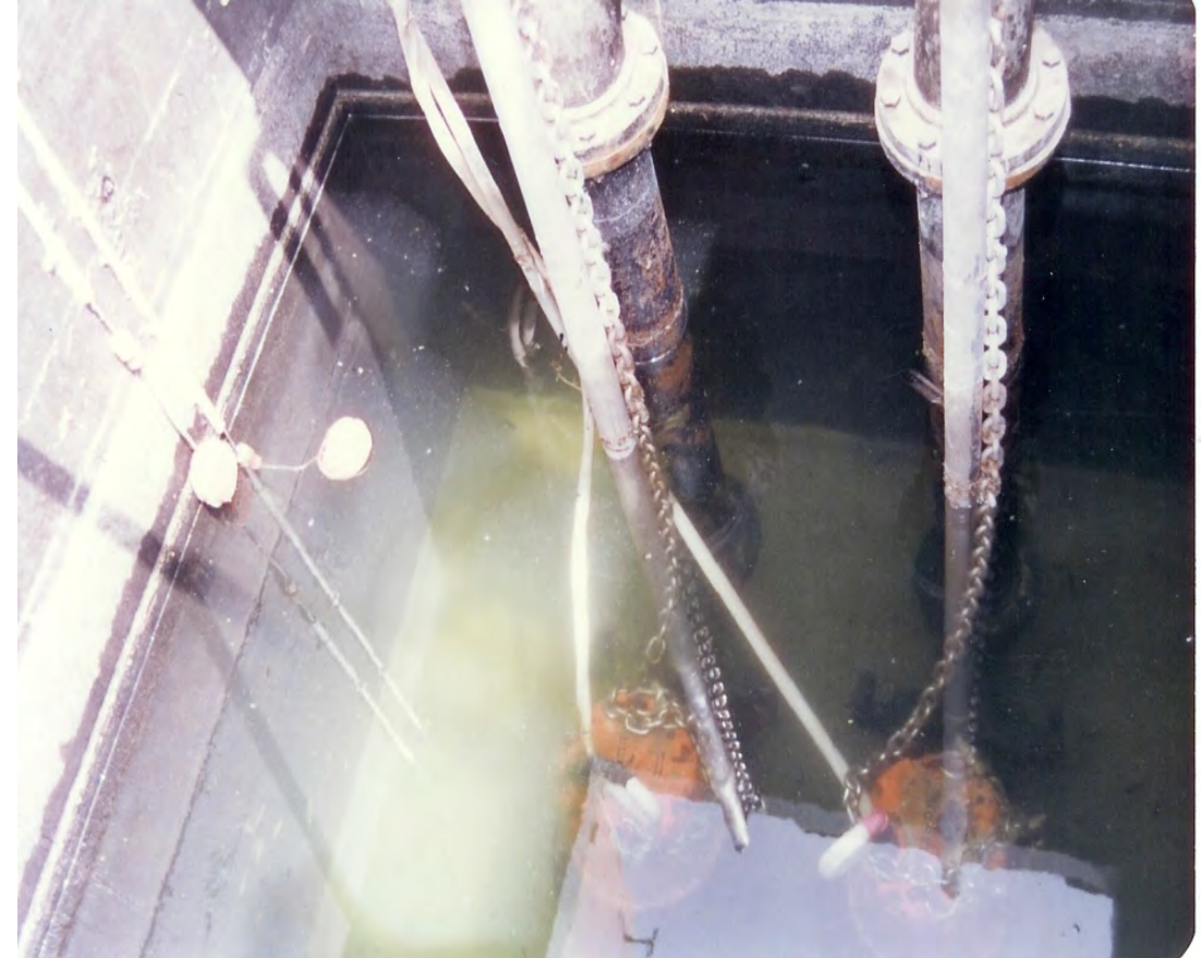
Secondary Treated Sewage Clarifier Pit Low to nil solid handling, high efficiency
