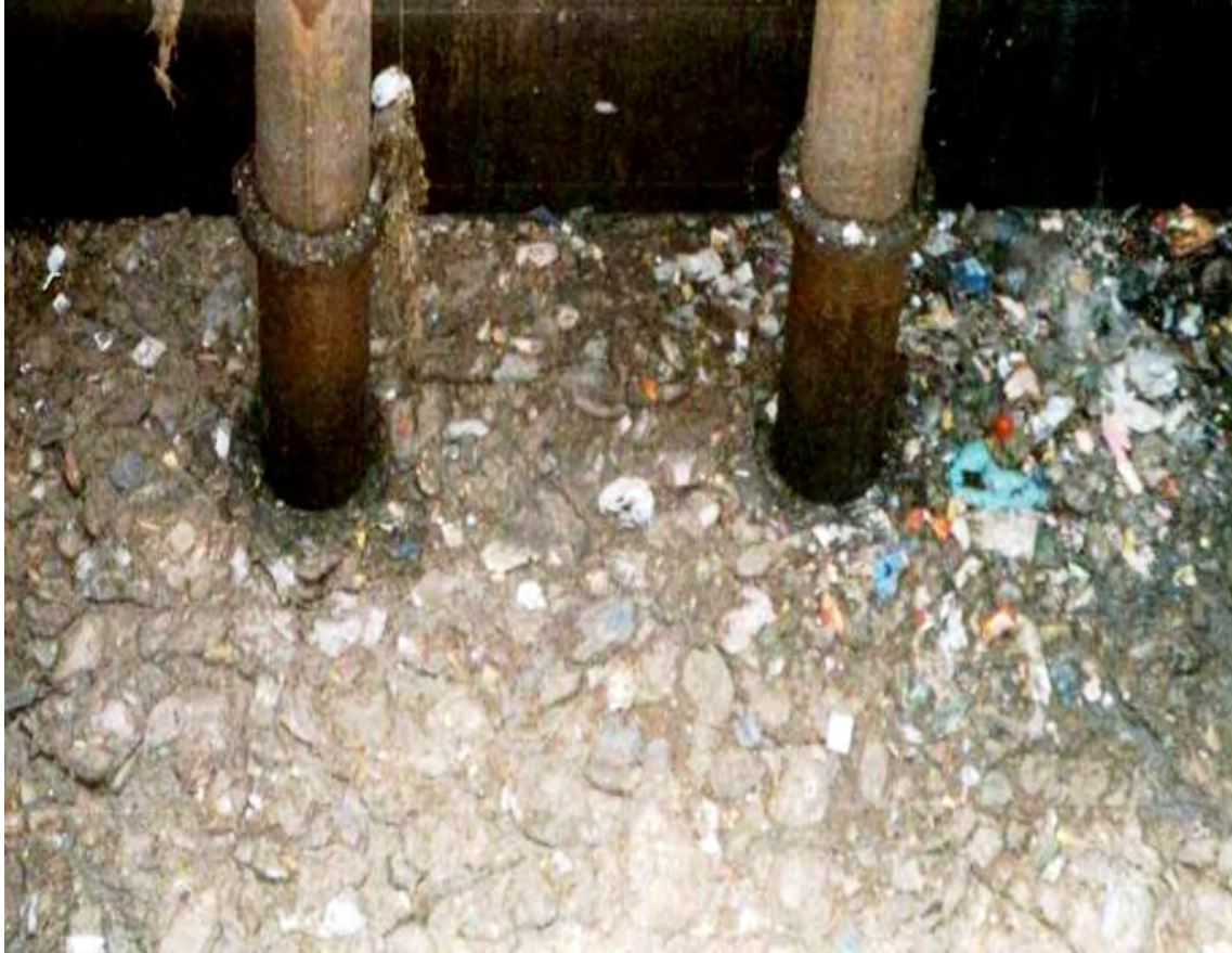
Raw Sewage Pumping Station Pit High solid handling, low efficiency
